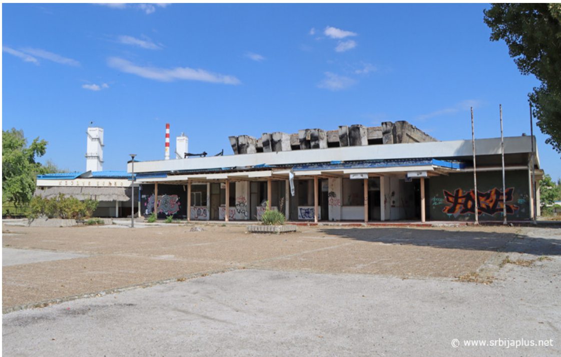
Figure 12. Bor Railway Station
