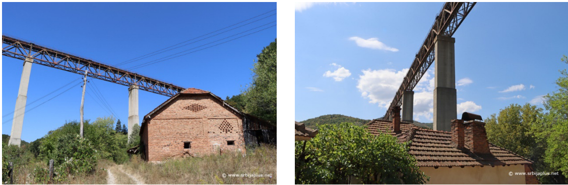
Figure 9. Viaduct Kriveljski Most
