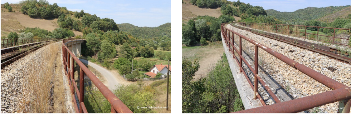
Figure 5. Viaduct Vlaole Selo
